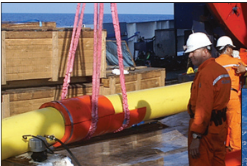
The riser being prepared for installation on board the installation vessel
